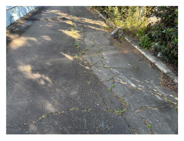
Photograph 5: Asphalt driveway with major cracking (890 & 896 Woodville Road)
